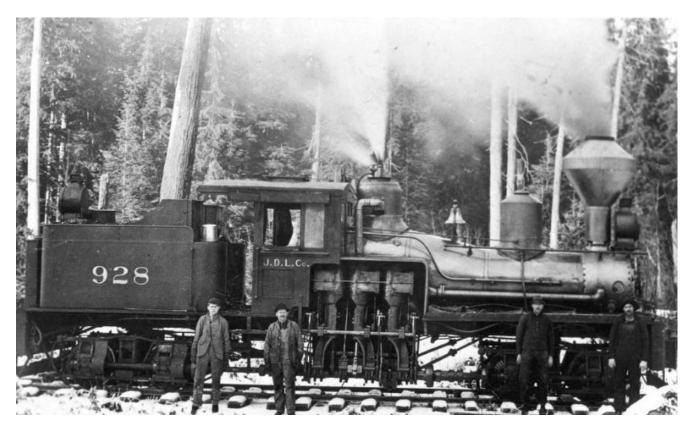
Most Shay locomotives sported three vertical cylinders, placed on one side, and had a long boiler that was offset from the centerline of the engine. Some had two "trucks" (sets of wheels) like #928, and some had three, carrying extra-large loads of fuel. The drivelines and universals were a mechanical marvel.
